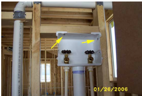
Looking @ washer hook up box – note nails used to anchor in place 10
