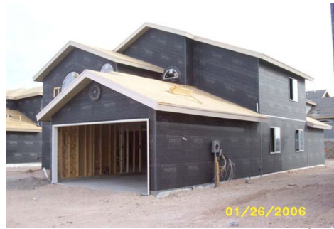
Looking south east @ west side of house 2
